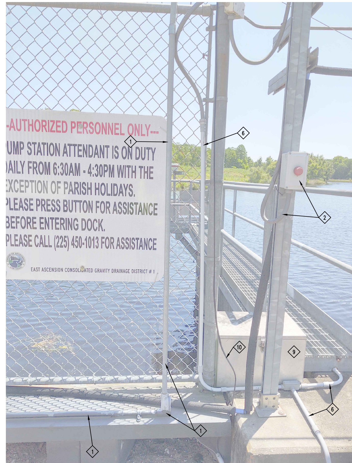
4 CONNECTION TO PUSH BUTTON STATION SCALE: N.T.S.
