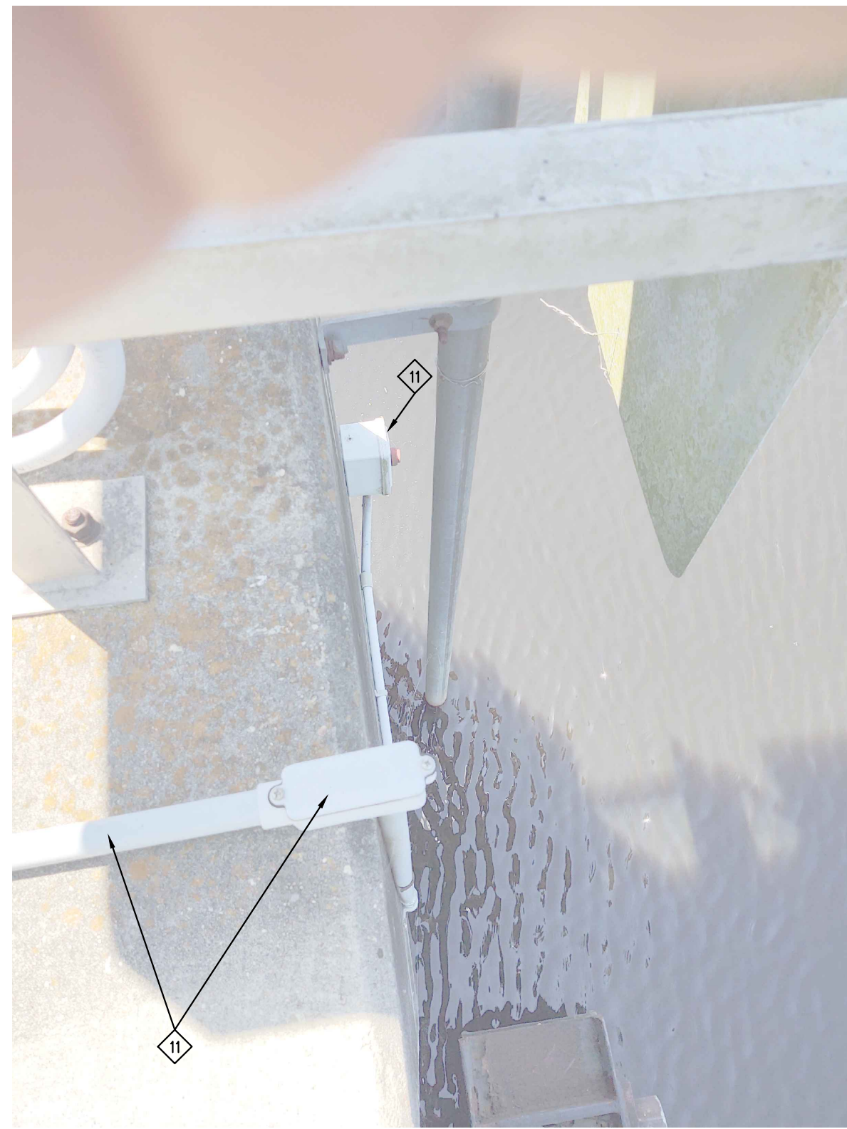
1 PUSH BUTTON STATION AT BOAT LOCK (TYP) SCALE: N.T.S.
