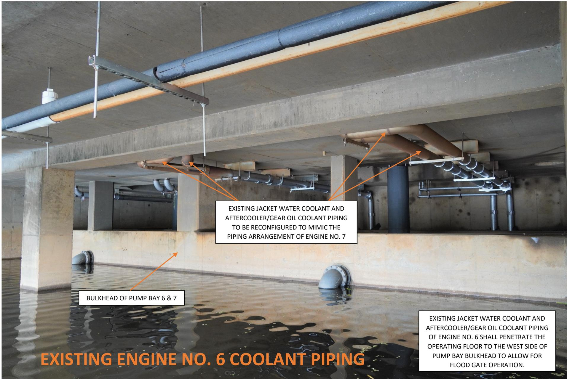
EXISTING JACKET WATER COOLANT AND AFTERCOOLER/GEAR OIL COOLANT PIPING TO BE RECONFIGURED TO MIMIC THE PIPING ARRANGEMENT OF ENGINE NO. 7
