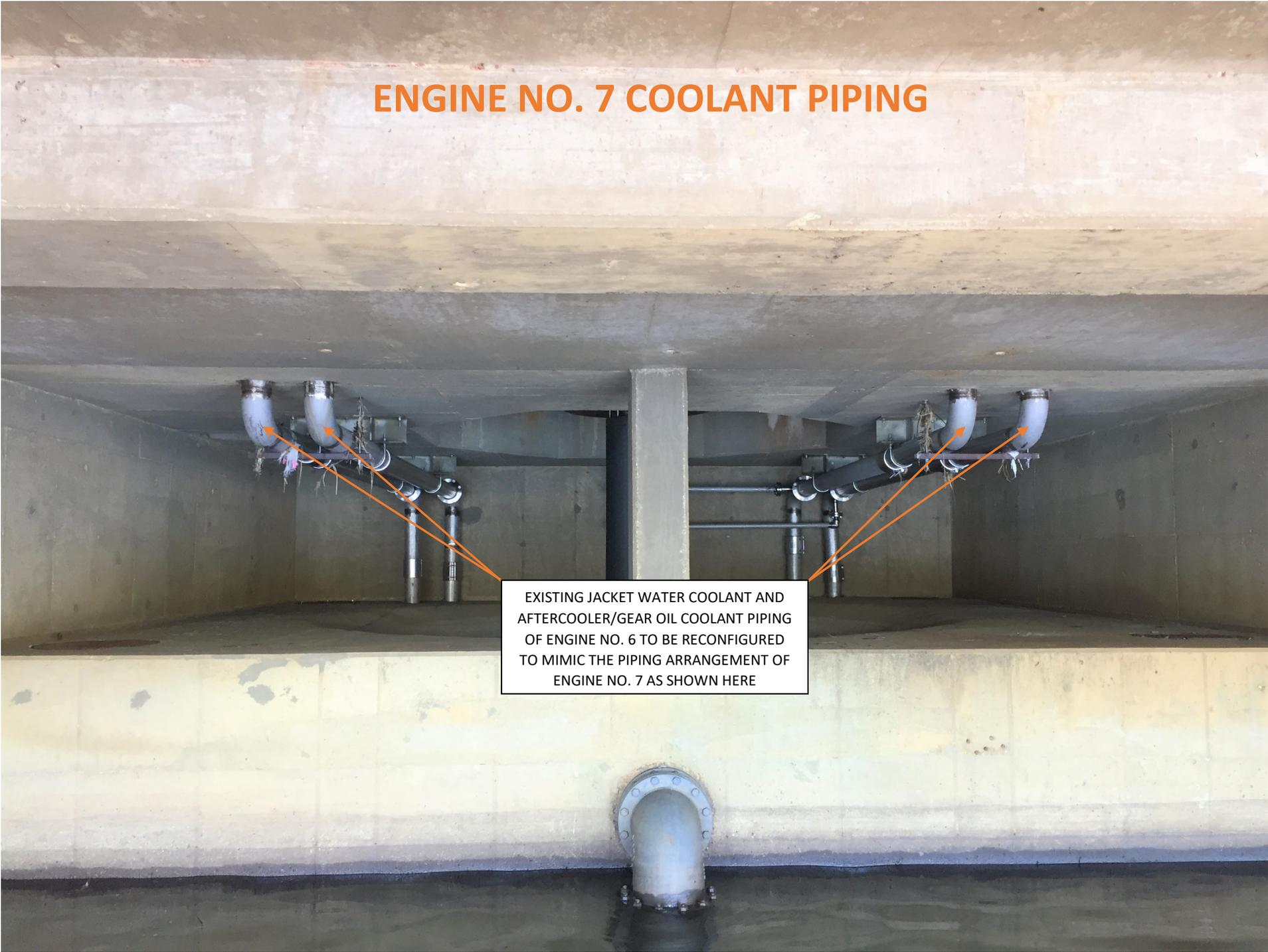
EXISTING JACKET WATER COOLANT AND AFTERCOOLER/GEAR OIL COOLANT PIPING OF ENGINE NO. 6 TO BE RECONFIGURED TO MIMIC THE PIPING ARRANGEMENT OF ENGINE NO. 7 AS SHOWN HERE
