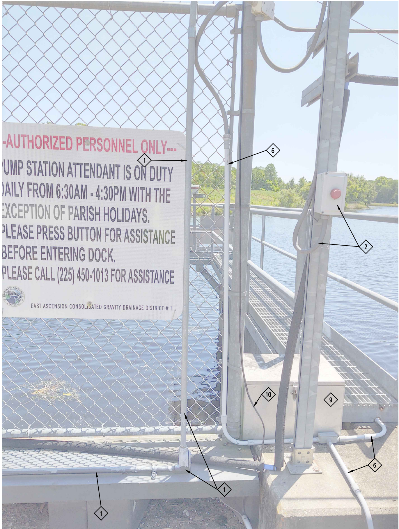
4 CONNECTION TO PUSH BUTTON STATION SCALE: N.T.S.
