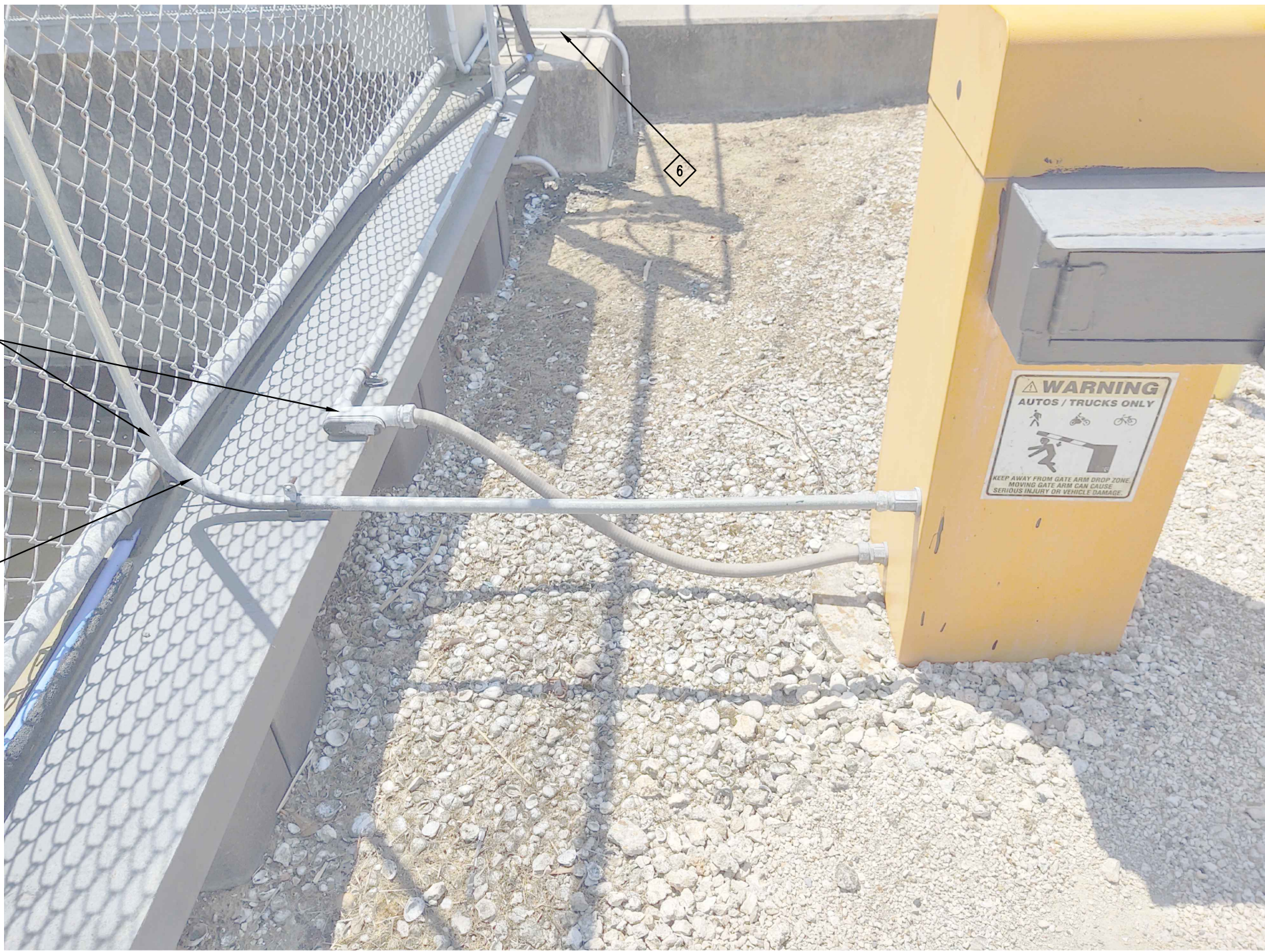
5 CONNECTION TO BARRIER GATE OPERATOR SCALE: N.T.S.
