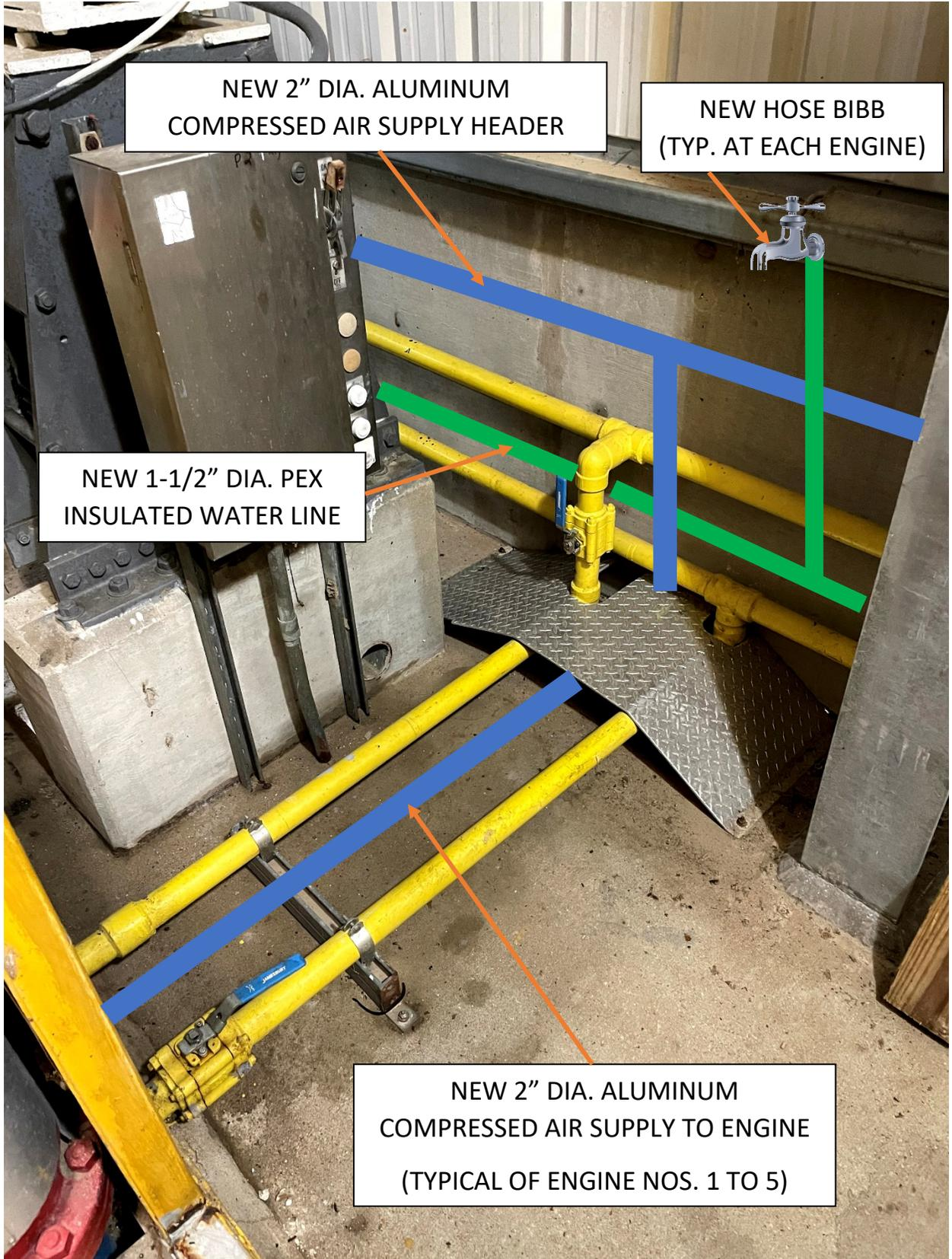
NEW 2" DIA. ALUMINUM COMPRESSED AIR SUPPLY HEADER
