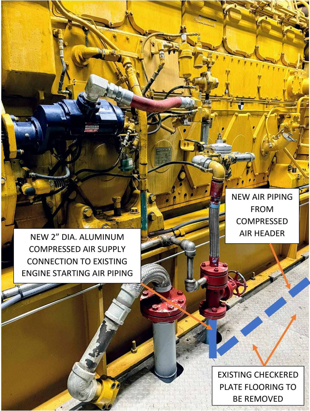
NEW 2" DIA. ALUMINUM COMPRESSED AIR SUPPLY CONNECTION TO EXISTING ENGINE STARTING AIR PIPING
